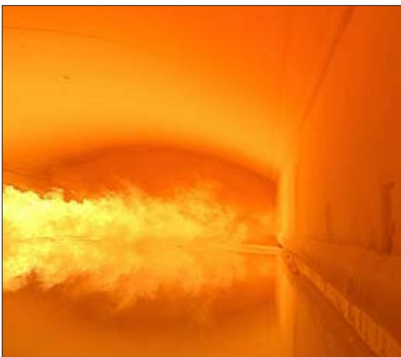
Flame analysis in a glass furnace
